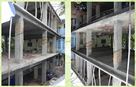
New block-under construction
