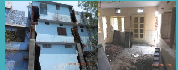
Putal Bai Complex – Refurbishment
