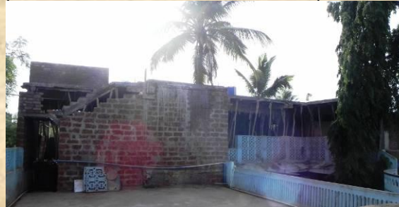
2 nd Floor Construction
