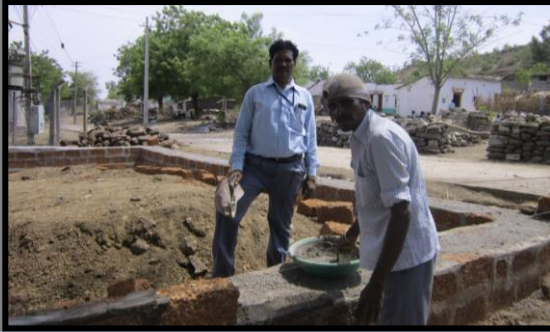
Kodampur Church basement construction.
