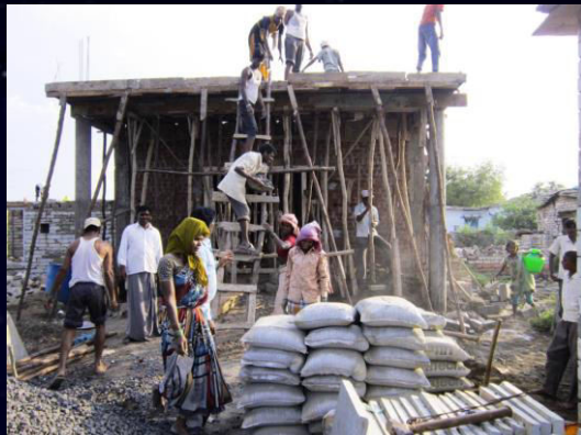
Goudanahalli Church construction almost completed
